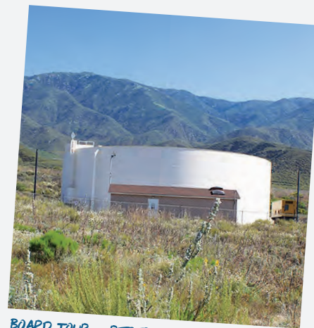
BOARD TOUR - RESERVOIR LOCATED IN THE ETIWANDA PRESERVE
